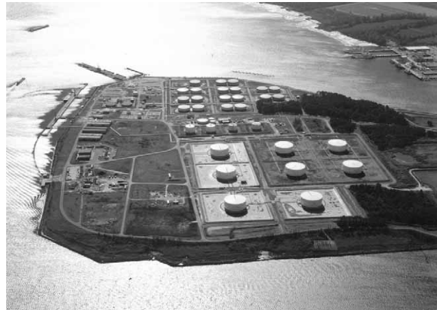
Fuel tanks at Craney Island
