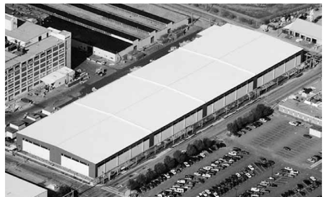
This general purpose warehouse, a 140,000-square foot defense distribution depot for the Navy is located at the Norfolk Naval Station.
