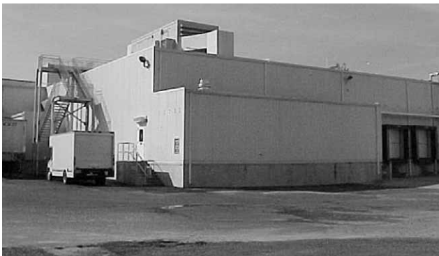
Gwaltney plant expansion at Smithfield Foods Inc.
