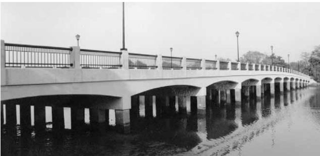
26th Street Bridge over the Lafayette River in Norfolk
